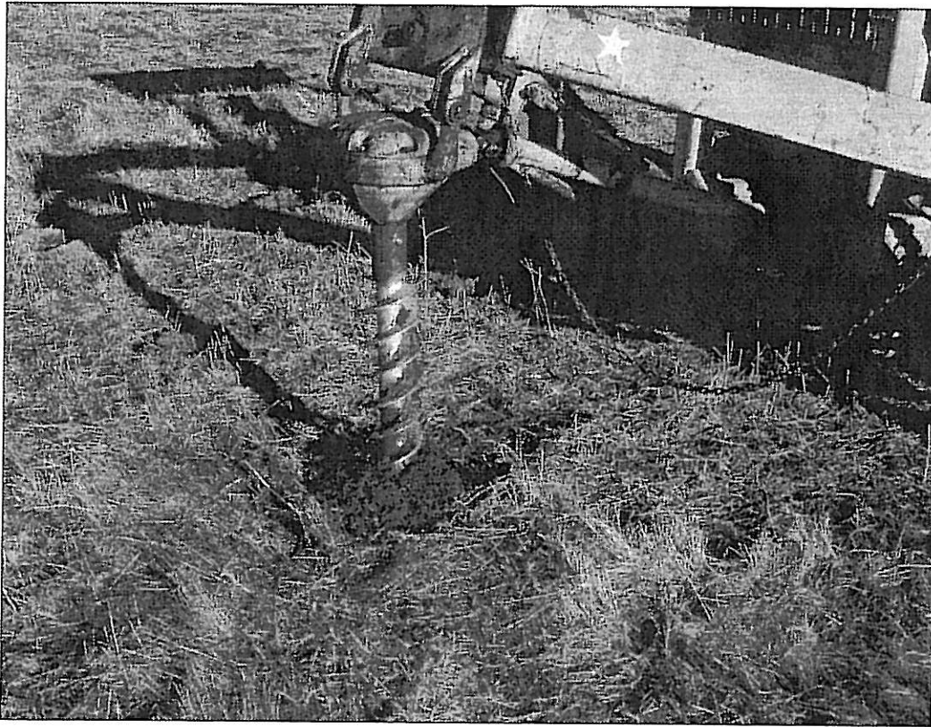
Figure 10. Tractor-mounted augers can be used to break through compacted soil.
